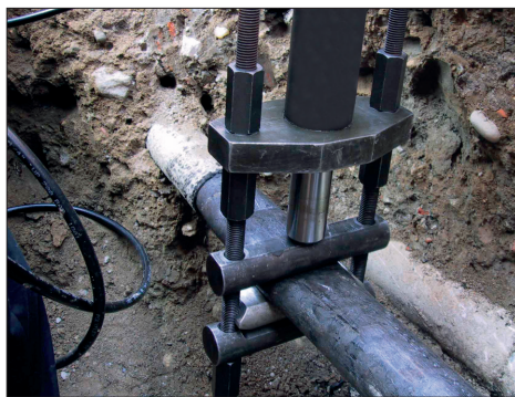
Pumping operation for pipe compressing
