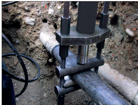
Pumping operation for pipe compressing
