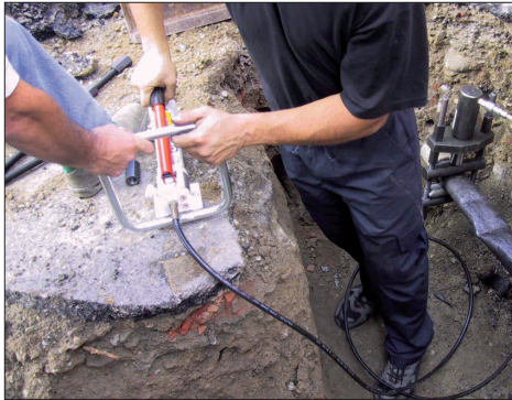
Pumping operation for pipe compressing
